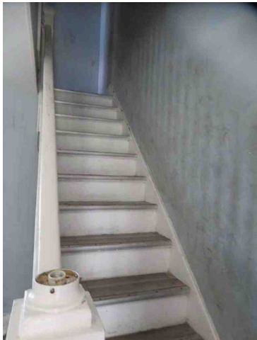
staircase to 2nd floor
