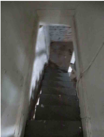
staircase to basement
